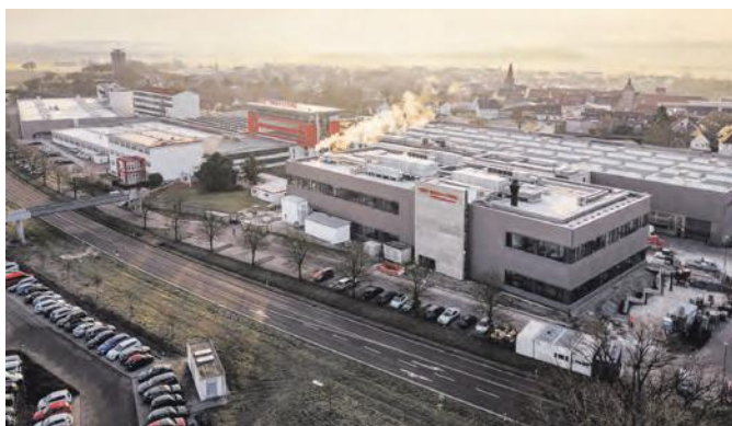
Bausch + Ströbel Headquarter in Ilshofen.
